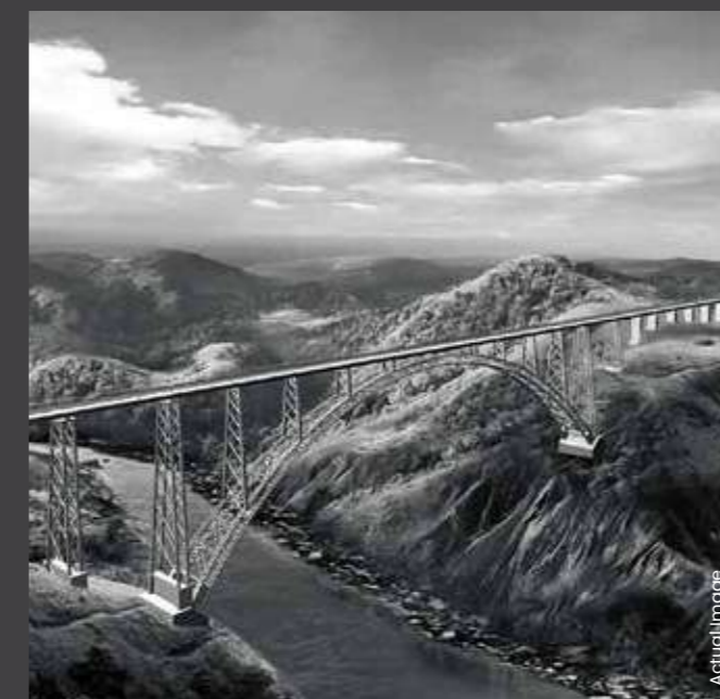
CHENAB BRIDGE, J&K
